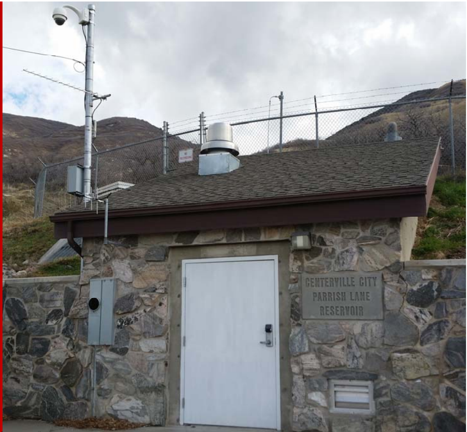
Reservoir and pump station in Centerville, UT
